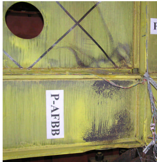
Fig. 5 RBS yielding and buckles at corner of panel following test of Specimen P
